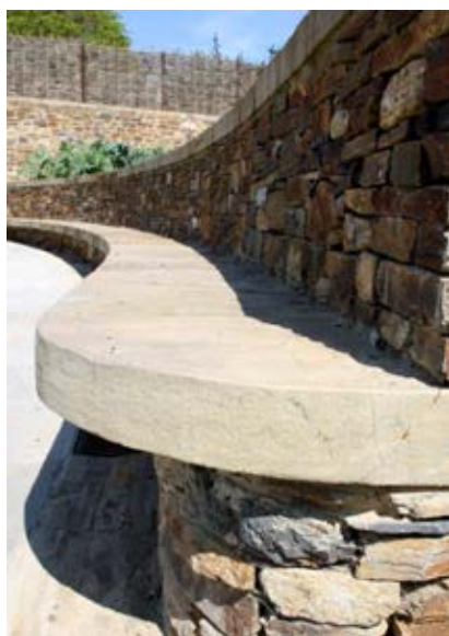
Walling and paving, Little Dartmouth
