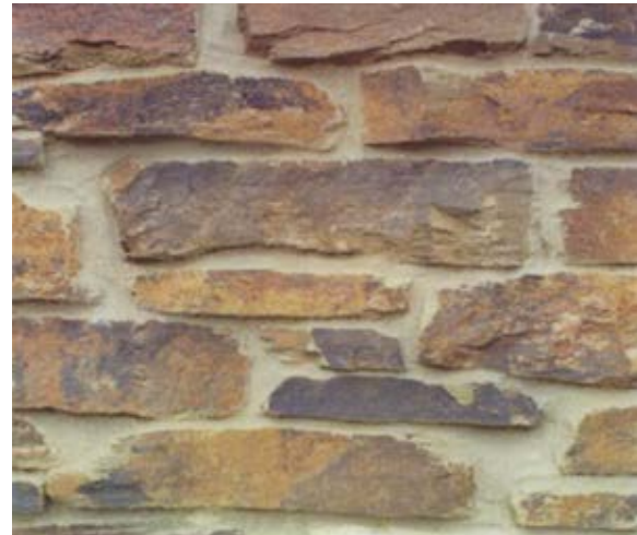
'Selected walling' stone – Yennadon Stone Note: parallel edges.
