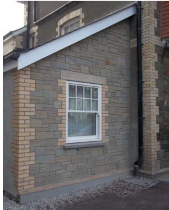
Recent extension in Tavistock built with Yennadon Stone as a Hurdwick replacement
